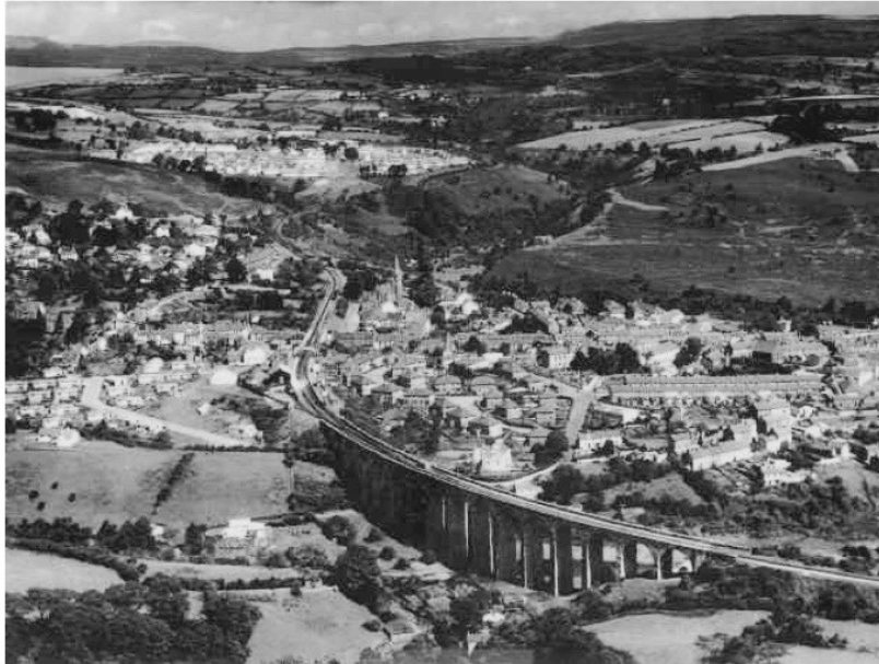
Aerial View of Cefn Coed showing Viaduct
